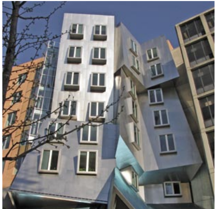
MIT’s new landmark structure, the Stata Center for Computer, Information and Intelligence Sciences in Cambridge, Massachusetts.
